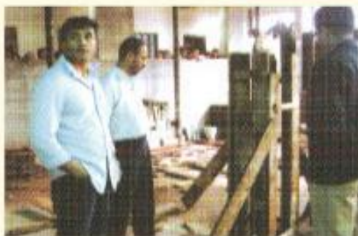
Job test for Shuttering Carpenter
